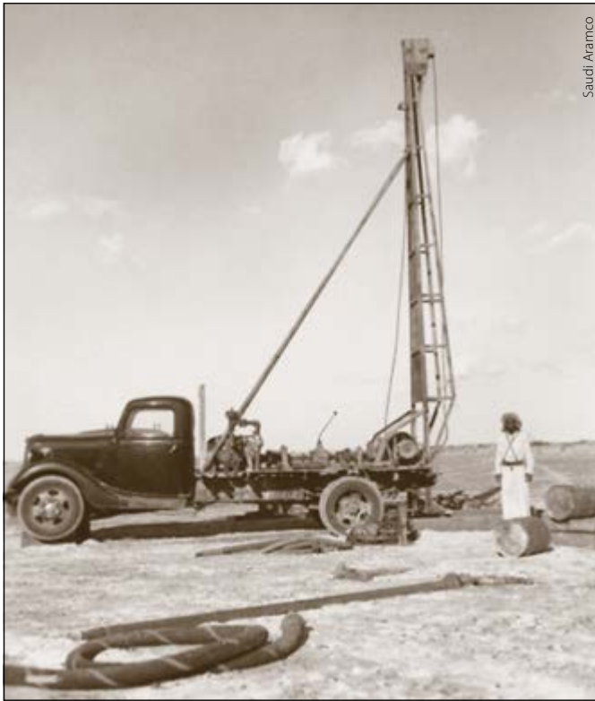
An early structure drill rig.
